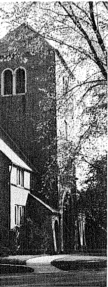
Dormitory Wing, South Entrance
