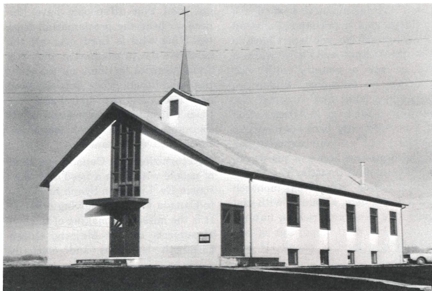
Exterior of St. John's Church at Wetaskiwin.
