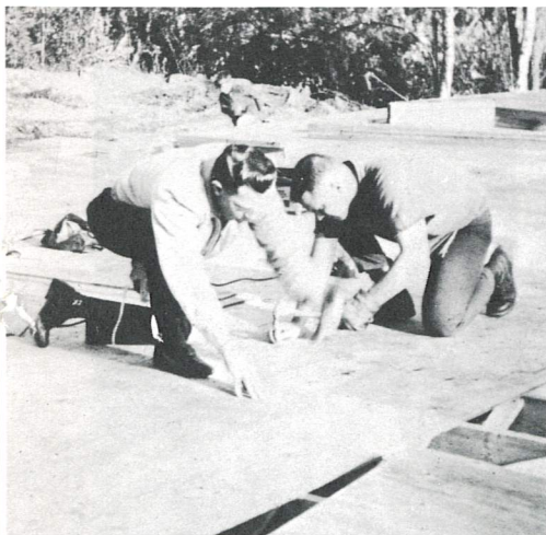
Building their church.
