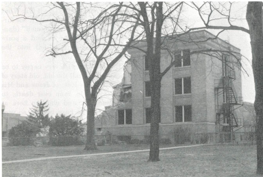
West Hall making room for the new.
