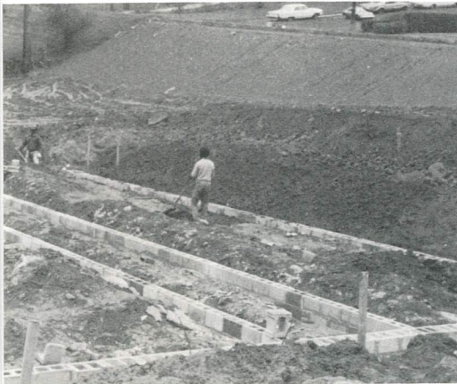
Preparing the foundation.
