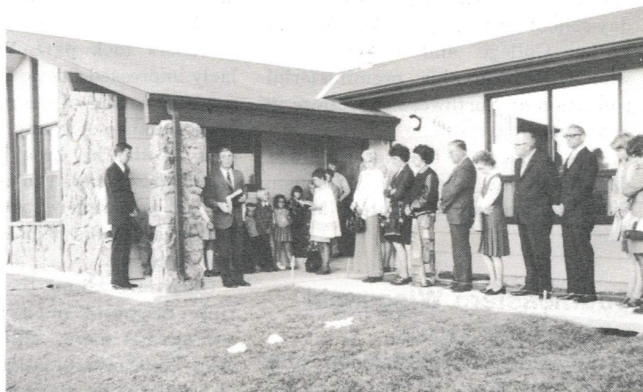
Parsonage in Fort Collins, Colorado
