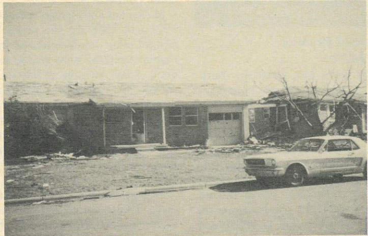
The Valleskey parsonage following the tornado
