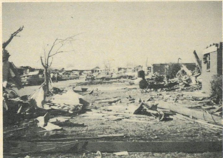
Typical of eight miles of the S.W. Parkway
