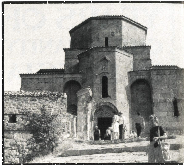
Partly ruined church near Mtskheta, Georgia.
