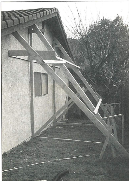
Supports propped up this house’s walls.
