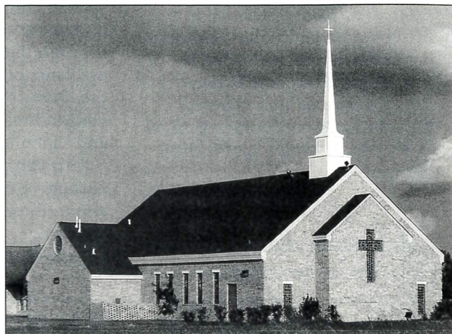
Builders for Christ helped build this new church for Prince of Peace, Houston, Texas.
