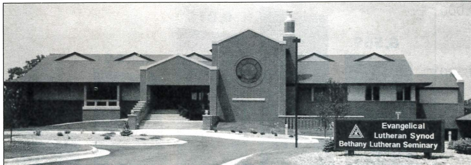
The new ELS seminary and synod office building houses administrative offices for the synod, and classrooms, offices, a library, and chapel for Bethany Lutheran Seminary, Mankato, Minn.
