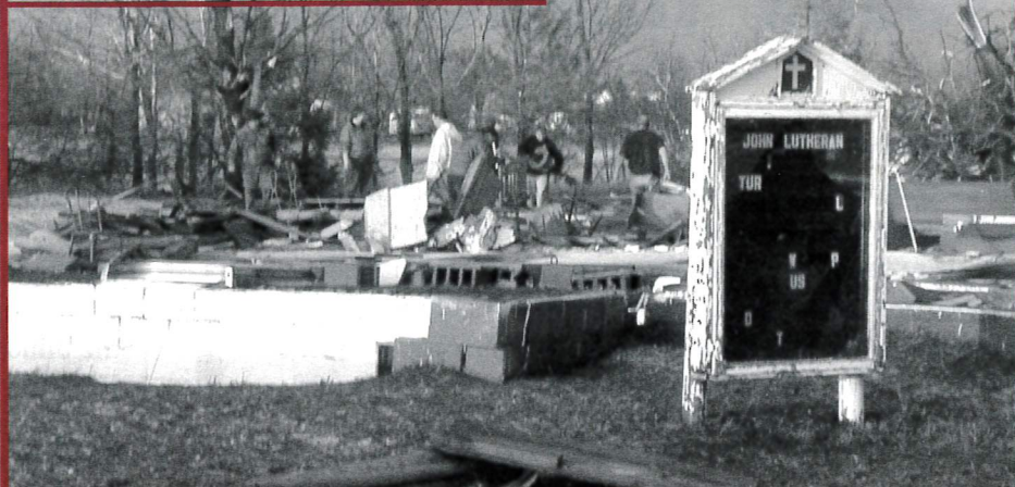
All that was left of St. John, Herrick, S.D., after an August storm was its basement, the front steps, and the church sign.
