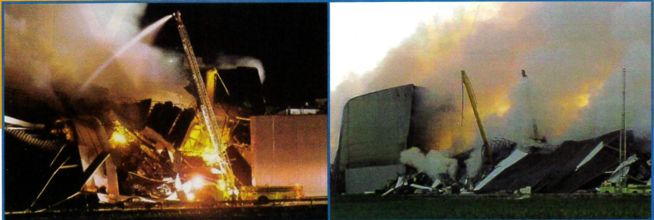
Quad/Graphics, the world's largest privately held printer, produces a variety of print materials, including Newsweek and Sports Illustrated magazines. A paper storage facility in Quad/Graphics' Lomira, Wis., plant collapsed and started to burn on July 12, 2002.
