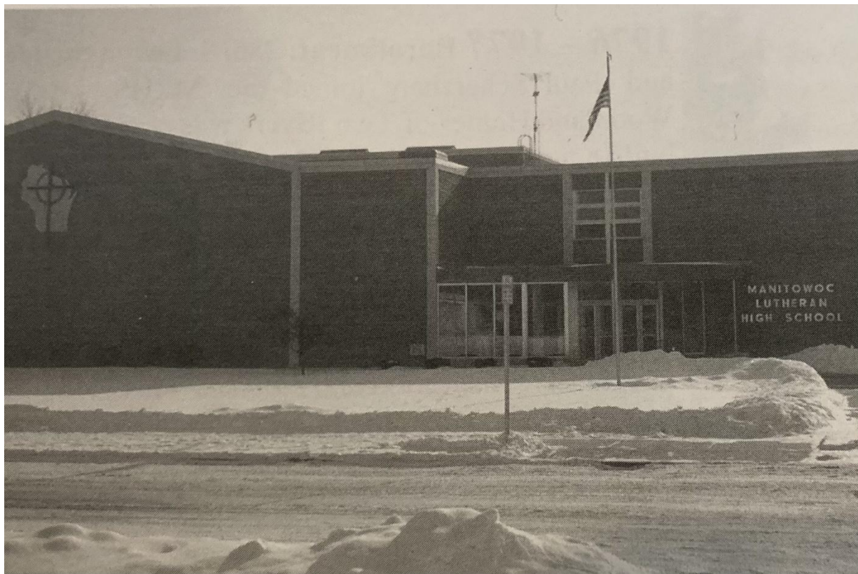
Newly constructed school building.
